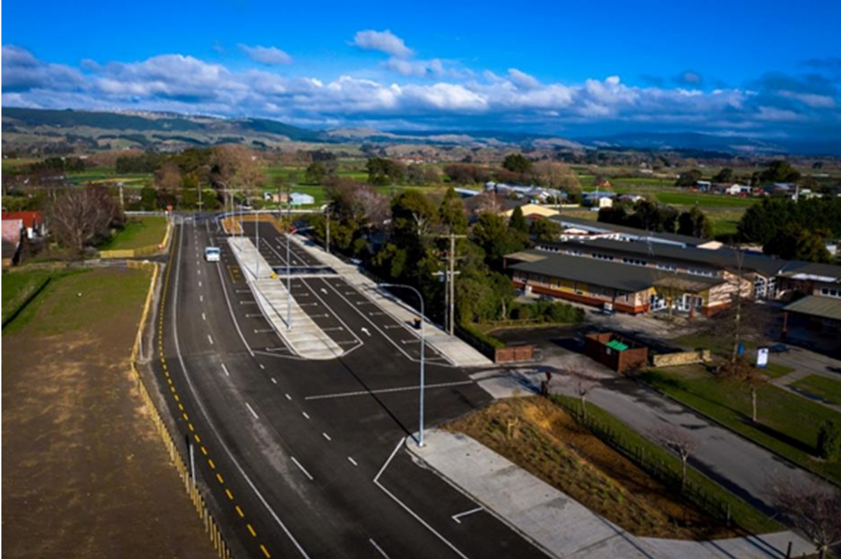
Figure 3 - Stoney Creek Road Safety Upgrade Project
