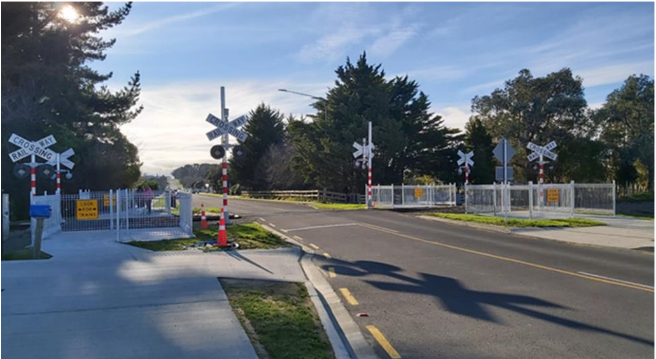
Figure 1 James Line – Railway Crossing Safety Upgrade
