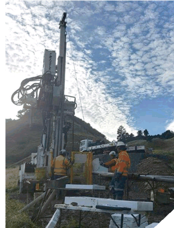
The crew at Te Oreore site drilling boreholes and installing groundwater monitoring devices, deep within the landslip area
