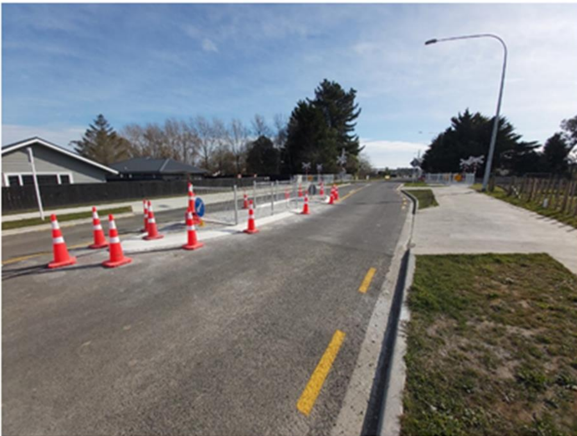
Figure 2 - James Line Pedestrian Refuge
