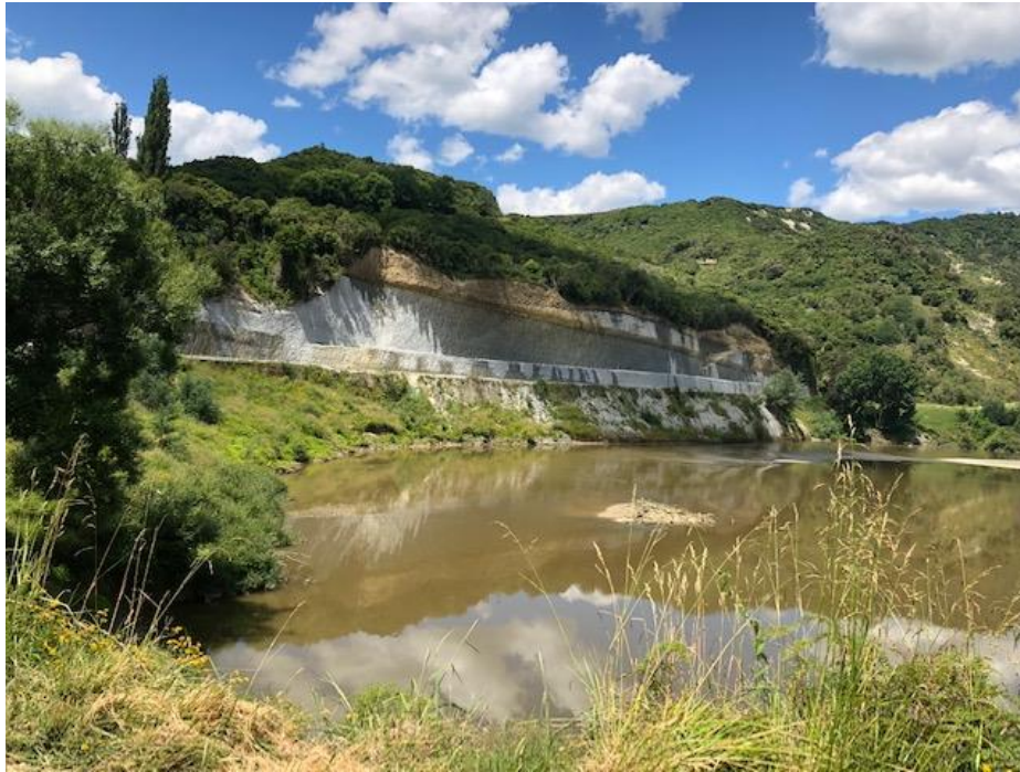
Photo: Taken standing on the August 2018 Jerusalem dropout, looking over to the June 2015 completed repair
